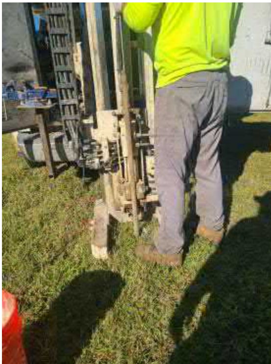
Photo 3: Representative view of drilling procedure
